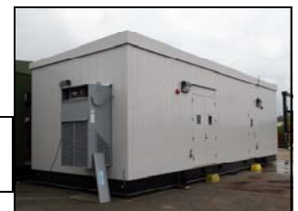
Modified bolted interlocked panel steel building to 6 psi.
