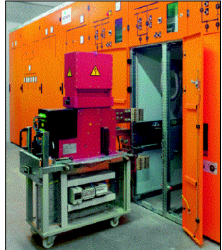
Typical DC switchgear traction arrangement.
